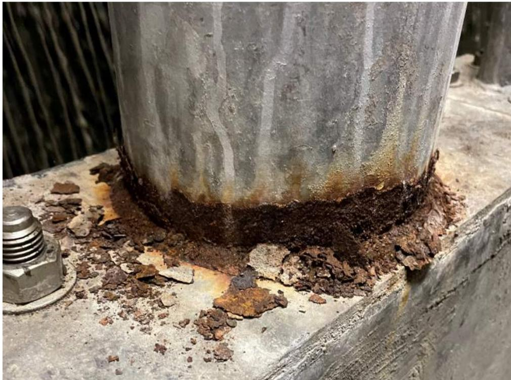
Photo 21: Rust and deterioration at column baseplates
