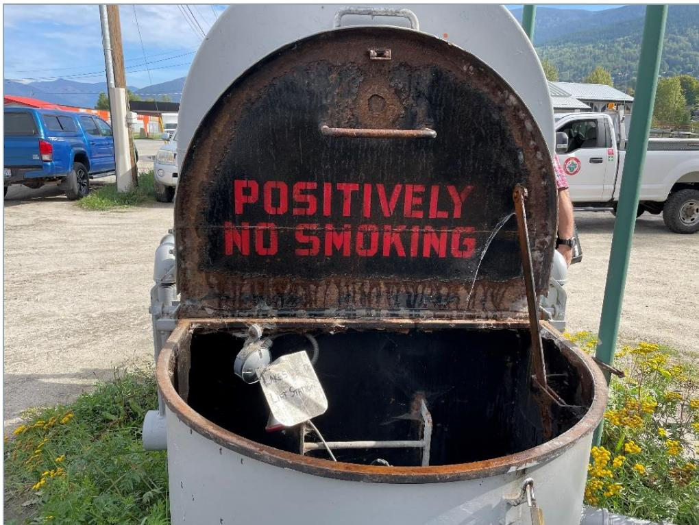
**Figure 2.2** Lakeside Drive Lift Station – Wet Well Hatch and Heat Lamp
