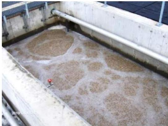
Figure 4 MMBR system in operation
