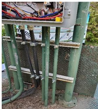
Unsealed conduits from the wet well below into the control panel.
