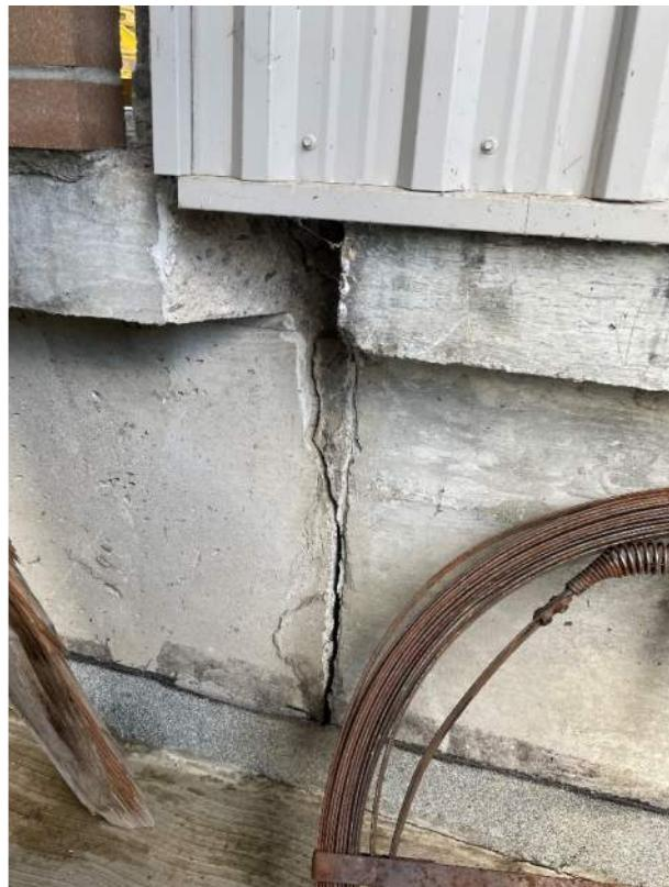
Photo 18: Cracking at east construction joint between the inlet and sedimentation tank 1
