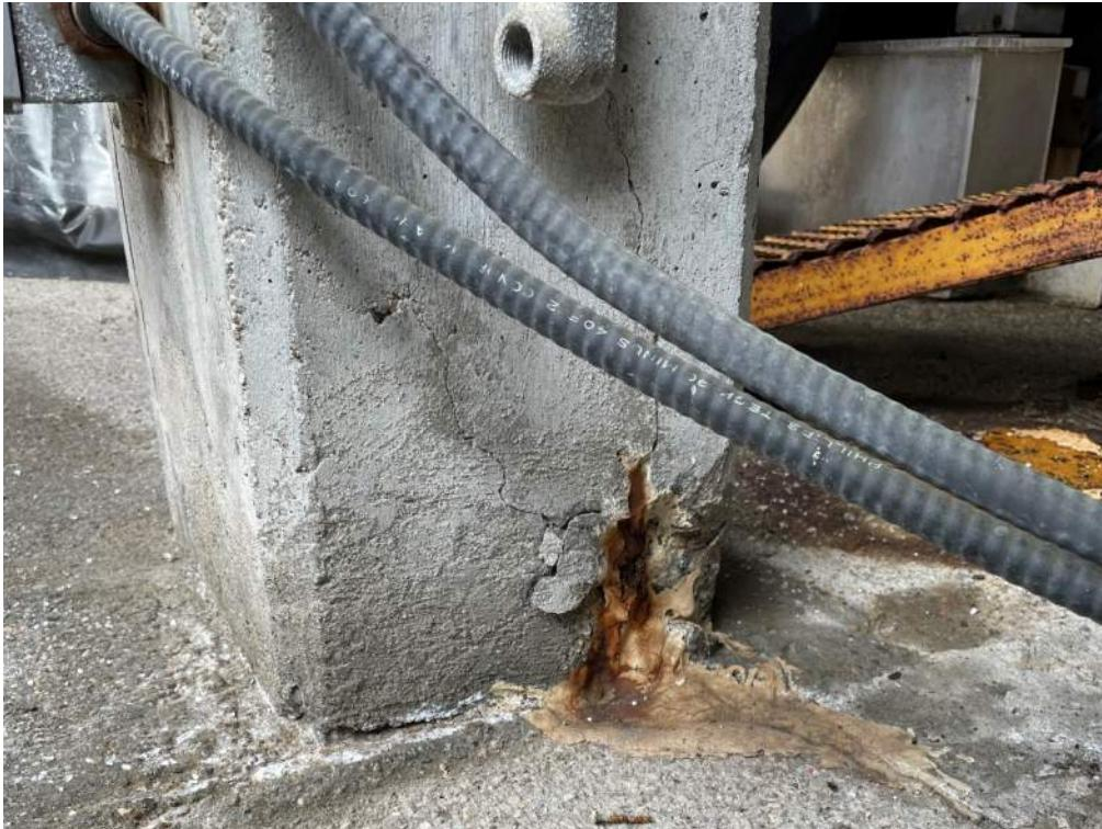
Photo 15: Cracking at column between grit tank and sedimentation tank 1
