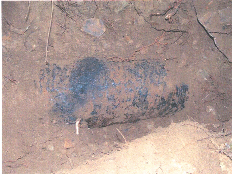
Image 13 – Water Main as Excavated
