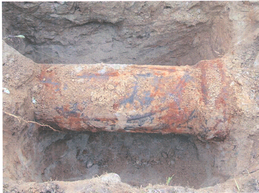
Image 3 – Water Main as Excavated
