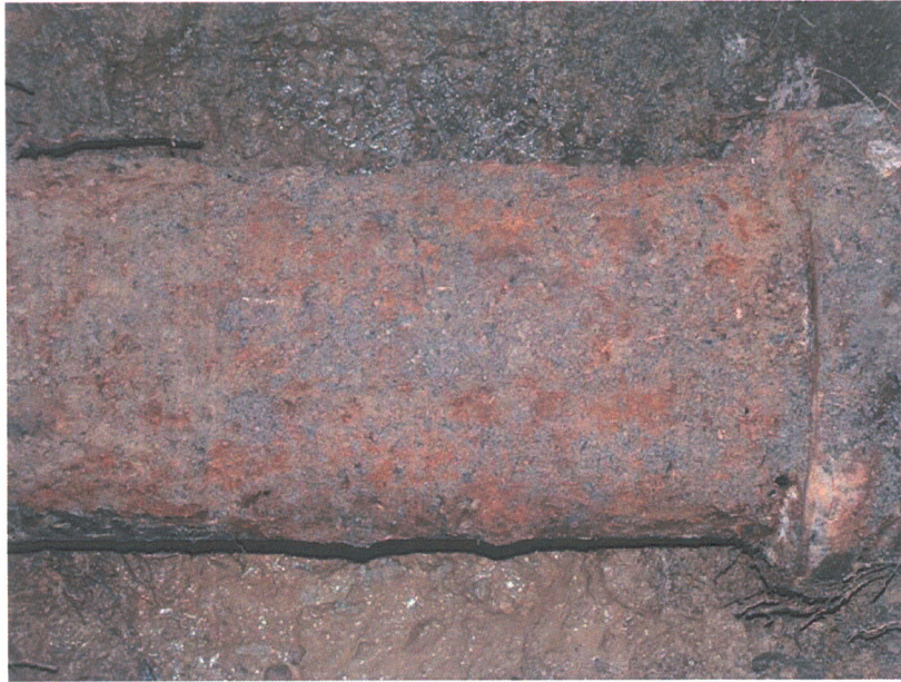
Image 9 – Water Main as Excavated
