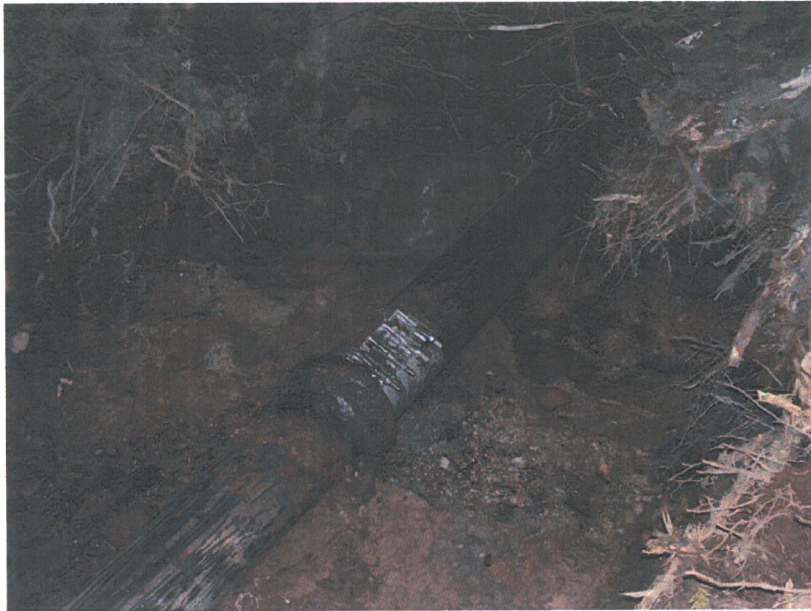
Image 7 – Water Main as Excavated
