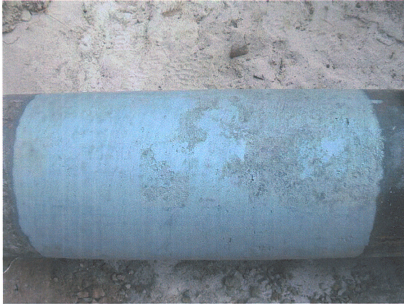
Image 19 – Water Main after Sand Blasting
