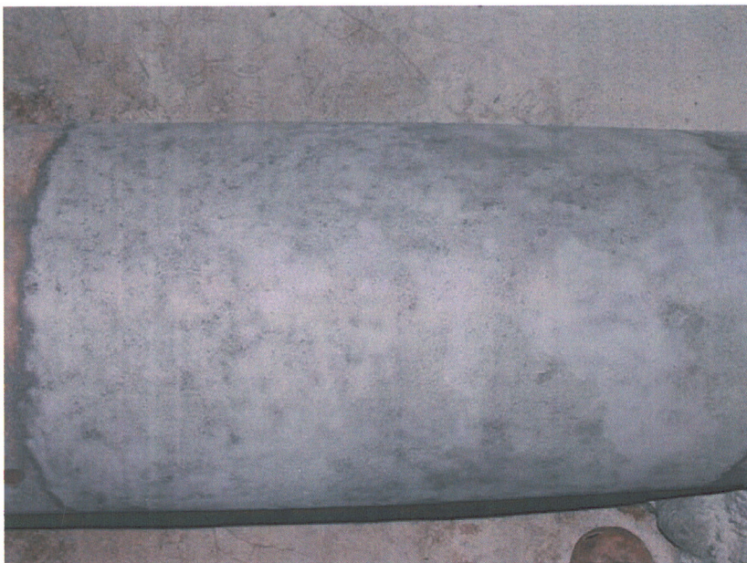
Image 2 – Water Main after Sand Blasting
