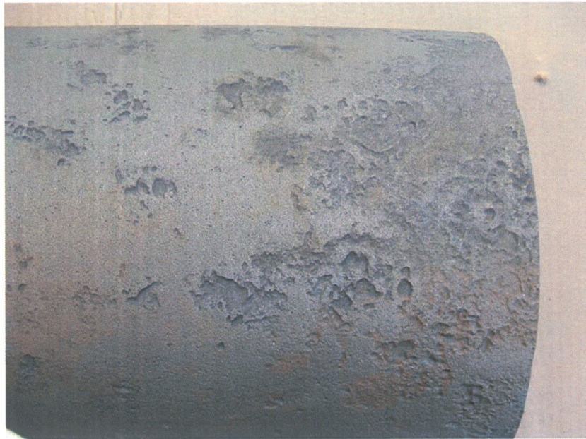
Image 27 – Corrosion Pitting on Exterior Surface
