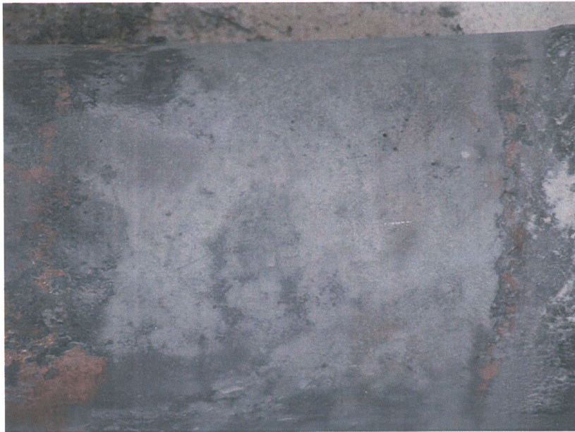
Image 10 – Water Main after Sand Blasting
