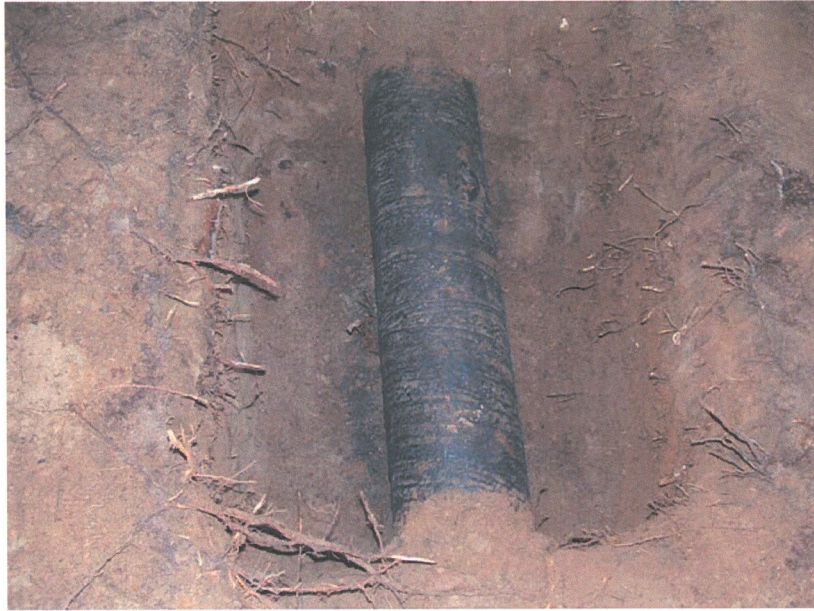
Image 14 – Water Main as Excavated
