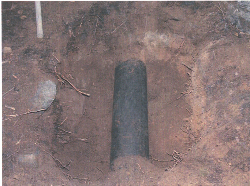
Image 16 – Water Main as Excavated
