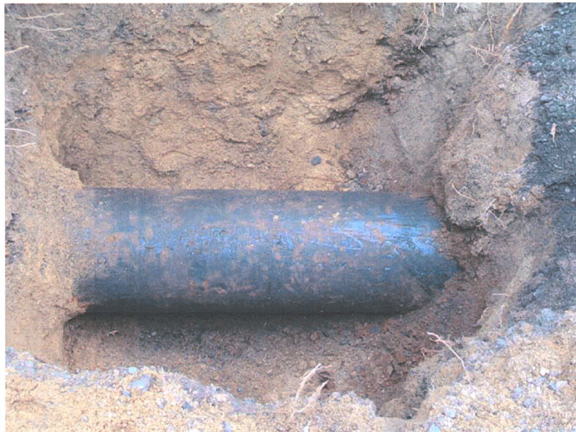
Image 5 – Water Main as Excavated
