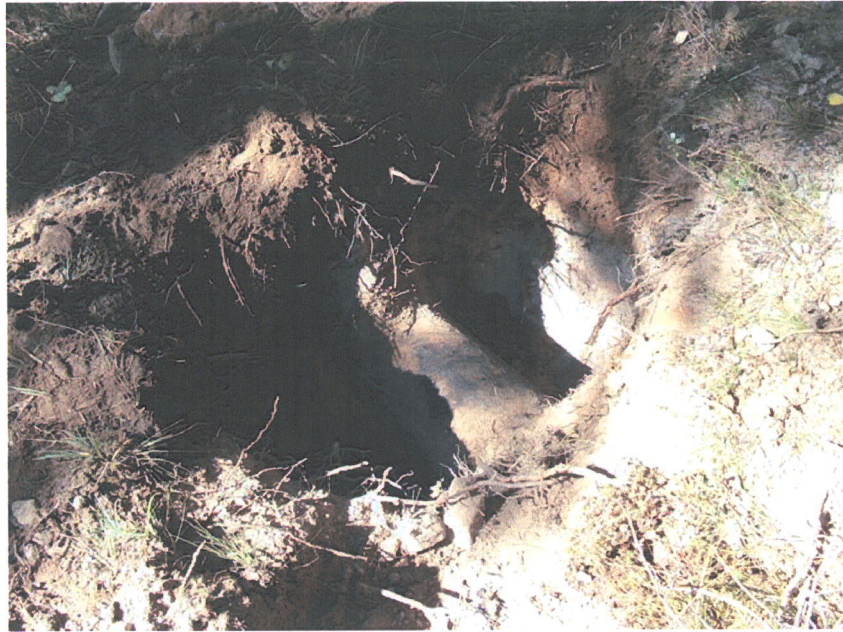
Image 12 – Water Main as Excavated
