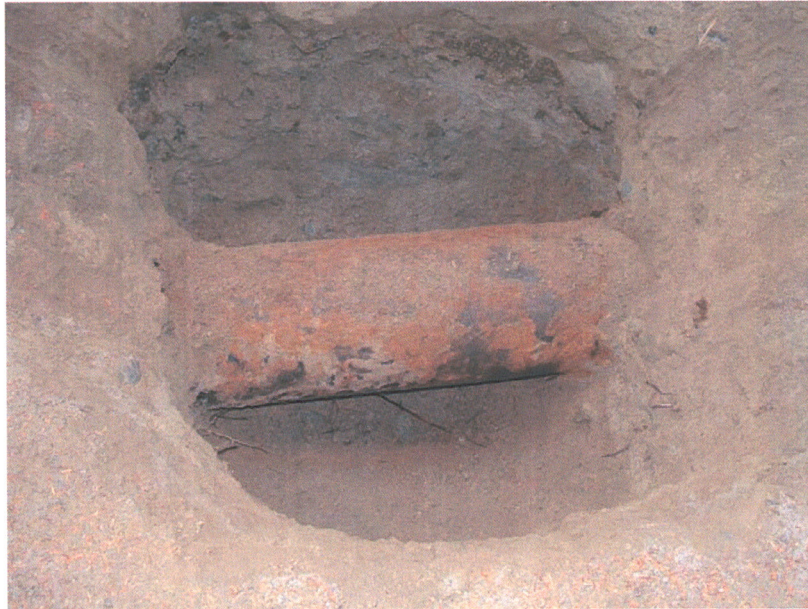
Image 1 – Water Main as Excavated
