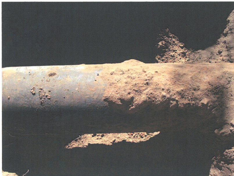
Image 18 – Water Main as Excavated
