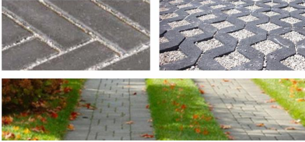
Examples of permeable parking (Credit: City of New Westminster)
